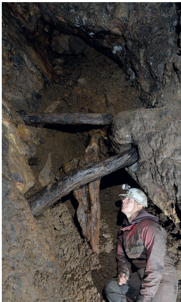
Figure 5: View of the supports in Chamber 2 of the medieval Alter Mann Victoria mine. Photo: P. Thomas, DBM.
