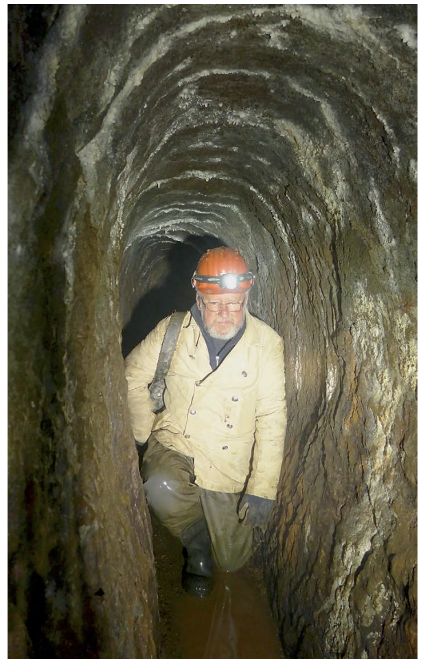
Figure 8: Cross-section of the gallery with balloon-shaped profile in the Stollen Mittlerer Sonnenberg Photo: R. Golze.
