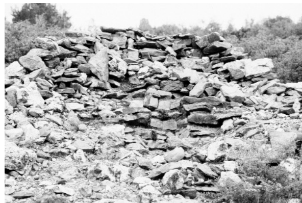
Fig. 8: Protection wall around the shaft of mine LR 5.
